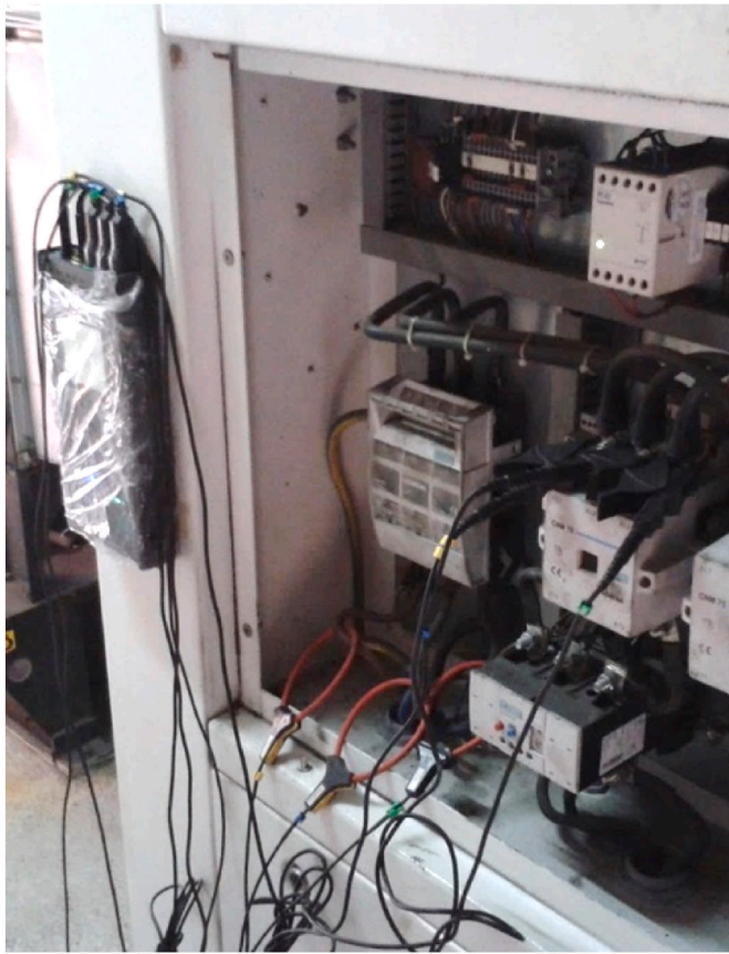
Fig. 3. Power demand measurement from the case study compressor.
